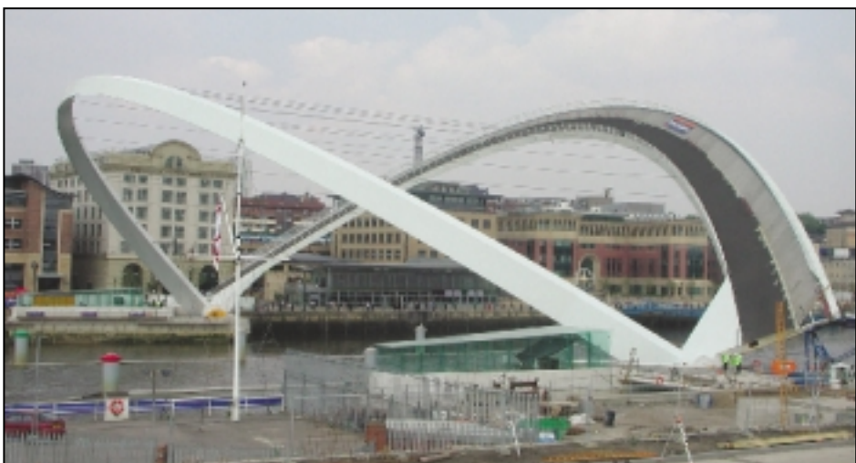
The Raised Bridge
